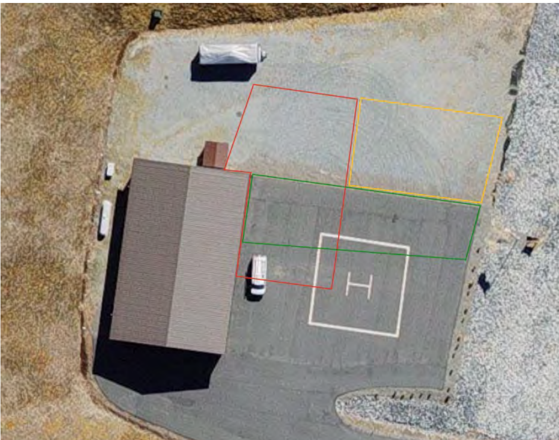
COVE CREEK – 08 (Zionville Fire Station #2)
